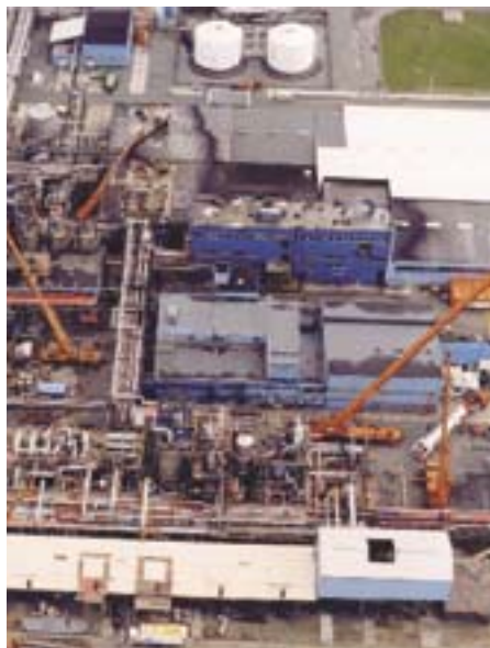
photos: kranen michielsens
