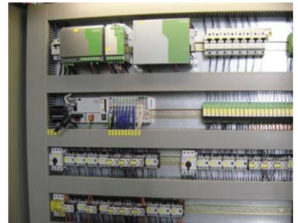
The ThinkIO - almost invisible among the electronic components. The compact rack PC hides to the left on the second top hat-rail.
