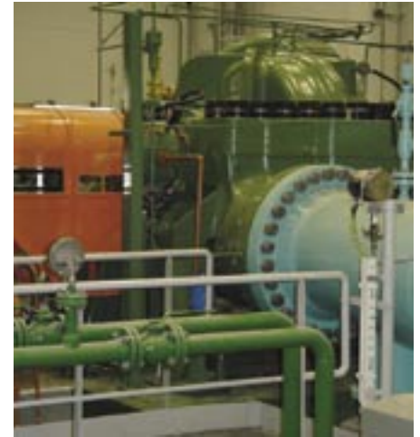
Fig. 3: Booster pumps (left) are much smaller than the main pumps. They provide the necessary suction pressure to ensure the smooth operation of the main pumps.
