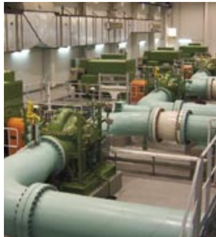
Fig. 3: Booster pumps (left) are much smaller than the main pumps. They provide the necessary suction pressure to ensure the smooth operation of the main pumps.
