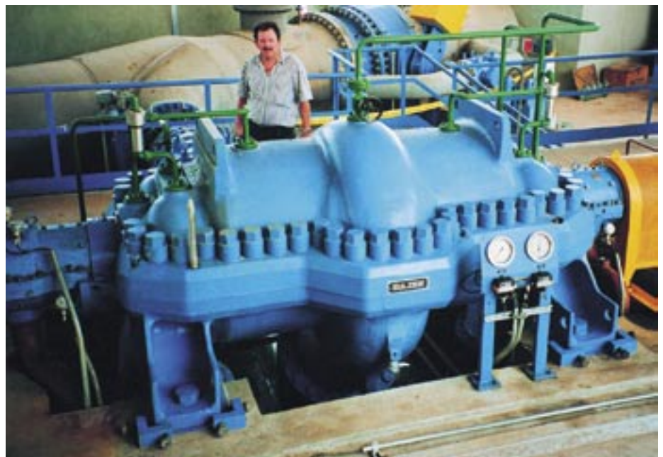
Fig. 4: The horizontally split casing facilitates maintenance. Suction and discharge connections are located in the lower part of the pump.
