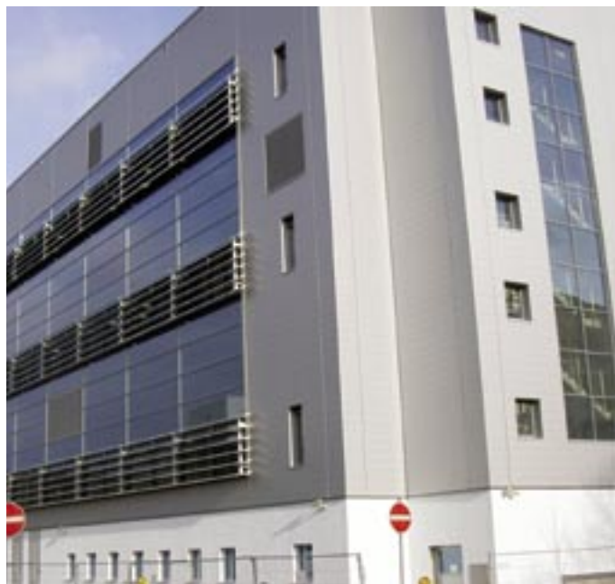
Spacesaving solutions also in building services were required in the extended building of GlaxoSmithKline Biologicals in the city centre of Dresden.
